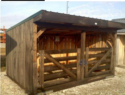
This is a good example of a pen for veterinary work as well as providing a shelter.
